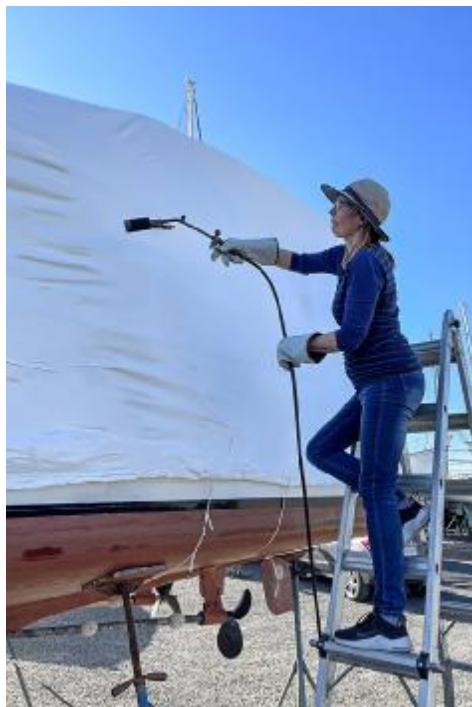
Erika using a heat-gun to shrink the wrap on Allure .
