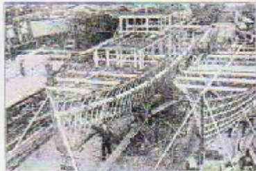
The above shows one of our 45-ft. COMPLETE FABRICATED HULL FRAMES IN BOX ready to be taken down and assembled. It is complete to the deck level of interior.
