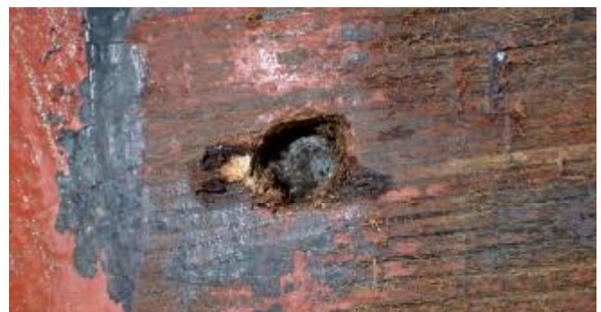
Boat nail. Sounded with 4# hammer and pin punch.
