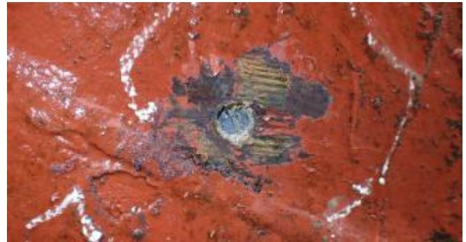
Galvanized, slot-head screw. Could not remove.
